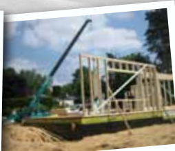
Timber Frame Work
