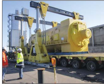
Turbine Lift and Load-in at Shipping Port
