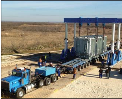
Transformer Installation with a Hydraulic Gantry
