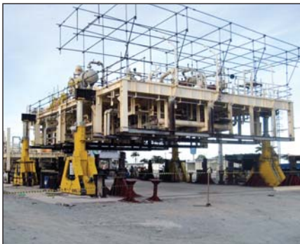
Assembling an Offshore Platform Oil Rig Module
